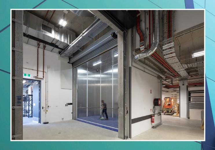
The newly completed HOTA Gallery required a custom designed hoist to assist in the movement of the gallery's iconic pieces. Southwell Lifts and Hoists, based in Camden in south-west Sydney designed, manufactured and installed the bespoke scissor art hoist with a 5 tonne capacity and a 5.9m x 2.9m platform.
